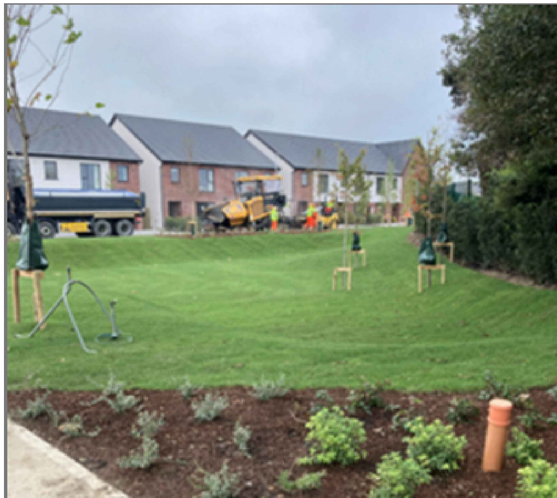
IMAGE 001 - OVERGROUND DETENTION BASIN EXAMPLE - PHASE 1 GRAYDON DEVELOPMENT
